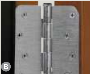
Heavy-duty stainless steel hinges resist corrosion and are standard in wind-borne debris regions.
